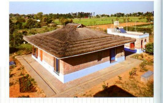
The house has a bamboo roof of *Bambusa balcoa* covered by a 30–35 mm layer of ferro-cement. For thermal insulation, the roof is covered with 30 cm of thatched straw. The walls are made of adobes (sun-dried brick).
